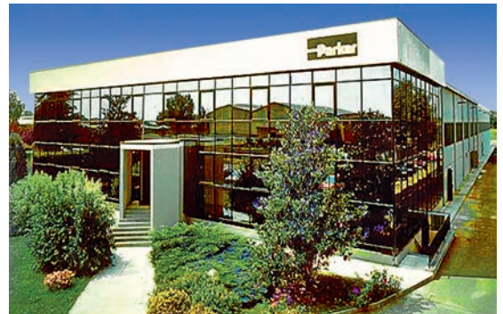
Gessate (Italy) Fluid Controls Solutions Europe
